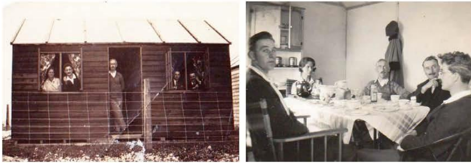
An example of the type of temporary accommodation that so exercised the local councils and freeholders. This was sited on plot 927 (29 The Parade), c. 1929. The interior shot of the hut demonstrates that they could be quite comfortable
