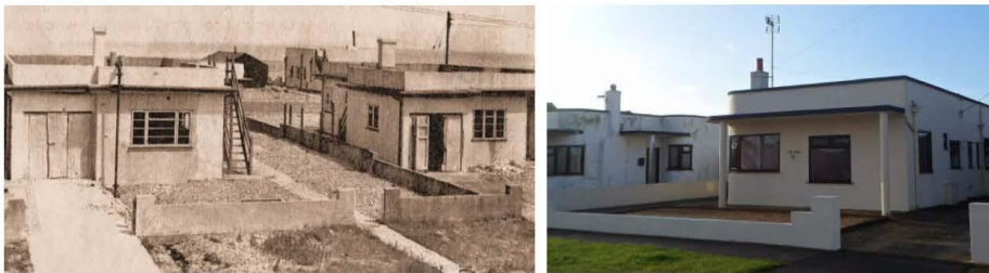
PLUTO bungalows in Leonard Road (Numbers 51 and 53), as built (left) and in 2013 (right). Opposite them (numbers 54 and 56) were PLUTO staff quarters
