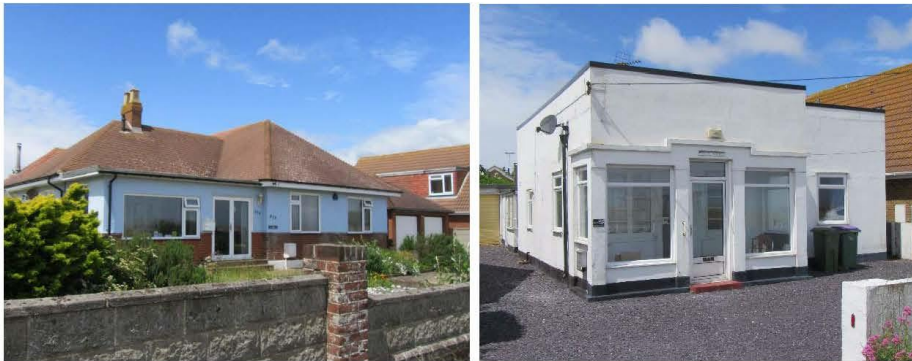
Anchorage (left) was purpose-built for PLUTO operations and accommodated two 10,000 gallon fuel tanks at the rear. Green Shutters (also in Coast Drive; right) was one of numerous properties to be adapted
